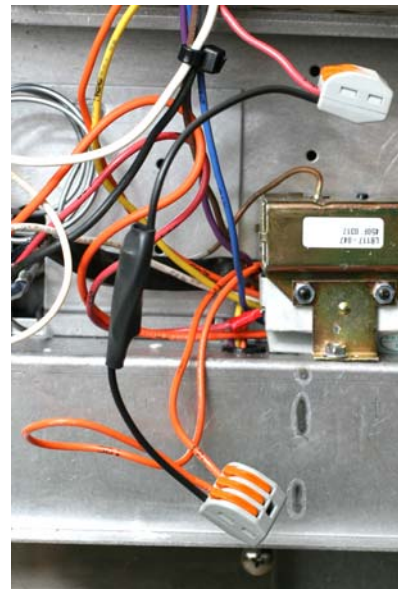
Figure 8: The new resistor is shown installed with provided connectors.
